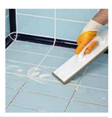
Always follow the same direction across tiles when applying the grouting material.
