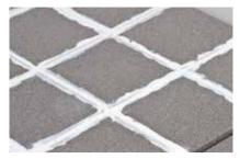
■ Remove the excess grouting material immediately using a rubber float moved diagonally (at 45°) across the tiles before it hardens. If moved parallel to the tiles the grouting material within the joints may be dragged from the joints causing a deformed grout surface. Always follow the same direction across tiles when applying the grouting material. If the joints are wide, particular care is required.
