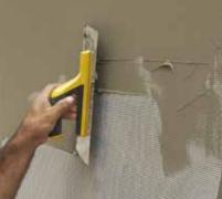
Adhesion and rigidity of the existing tile covering should be checked by tapping a hummer. Loose or poorly adhering covering should be removed and replaced by similar covering or the substrate should be reconstituted with a suitable repairing product. Before plastering onto existing tiles, surface adhesion should be improved for impervious the substrate with primers including thick fillings.
